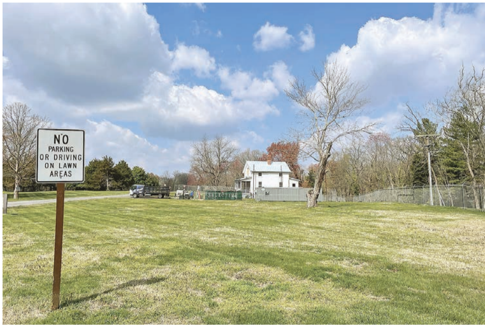
The house is now fenced off while the exterior is being stabilized.
